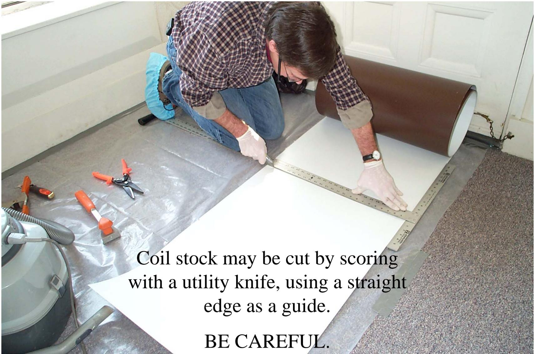
Coil stock may be cut by scoring with a utility knife, using a straight edge as a guide.
